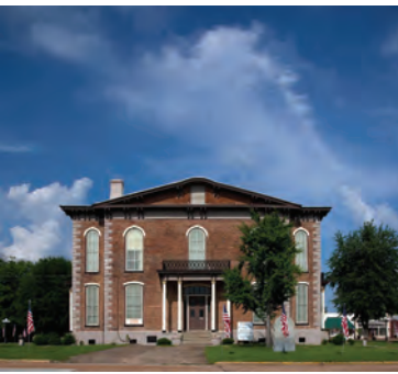
The Pickens County Courthouse in 1951, 1976, and 2010. Through the years, visitors continue to look for the Face in the Window. (Photos courtesy of the Alabama Department of Archives and History and the Library of Congress)
